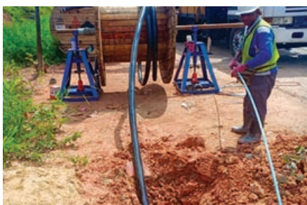
Power cable installation
