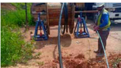
Power cable installation
